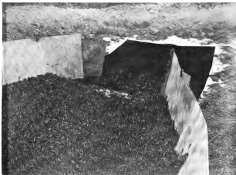
DRIVING SALTONAS INTO PITS.
